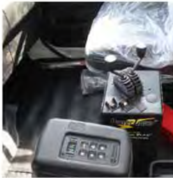
Inside air controls mounted in Power Tower
